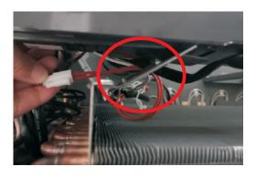
5. Disconnect the bottom tray heater cable from the original cable.
